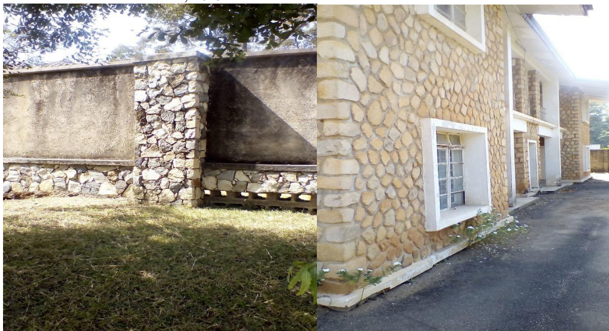
Plate xv: A mortared stone wall made from Limestone used for fencing at G.R.A. Jos. Source: Author's field work, 2019
