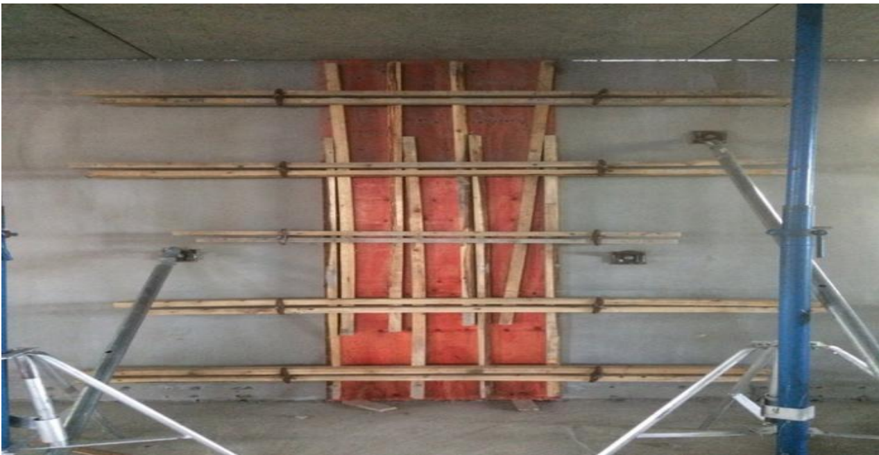
Fig. 7 Cast-in-site Connection between two Wall Panela
