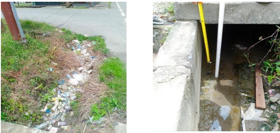
Fig. 4 Sedimentation in the drainage can block the flow.
