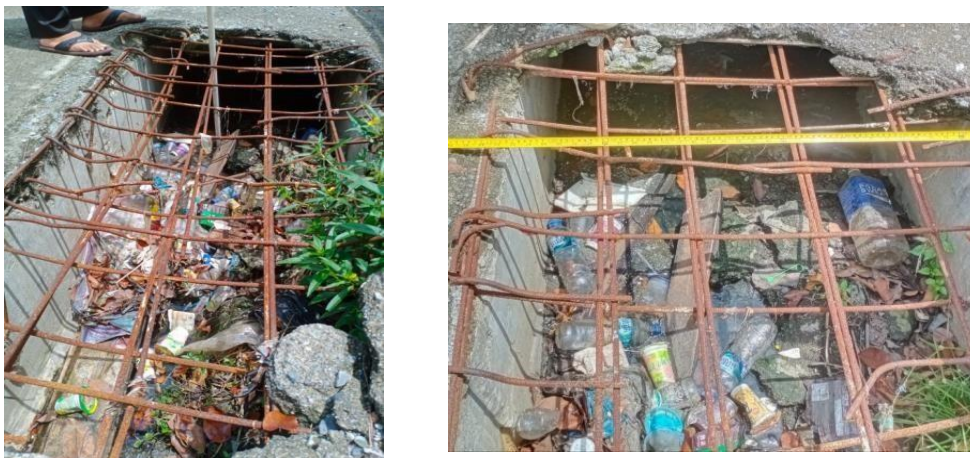
Fig. 3 There is much garbage in the drainage channel, and there is damage to t
